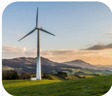
Wind and photovoltaic
